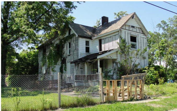
319 W MYRTLE: DEMOLITION
