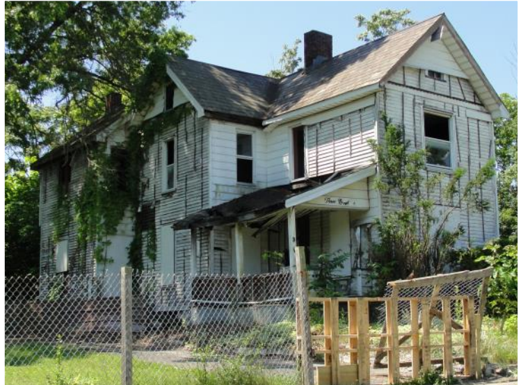
A blighted home in the Oak Hill neighborhood.
