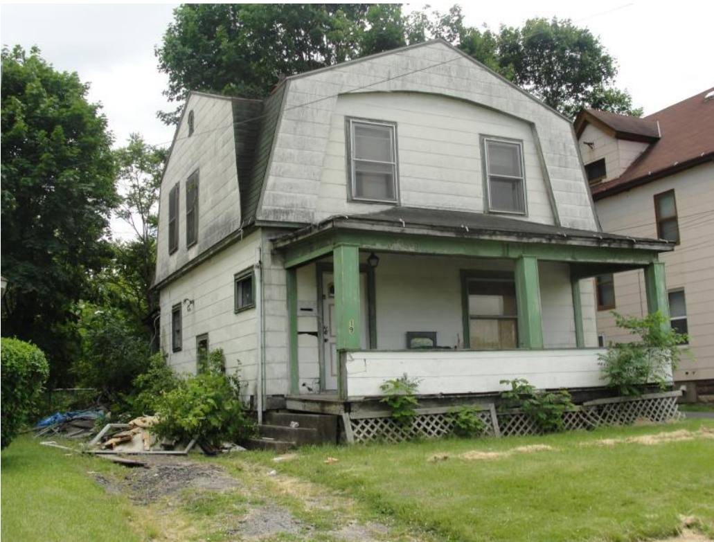
This blighted home in the Oak Hill neighborhood has a detrimental effect on the surrounding area.
