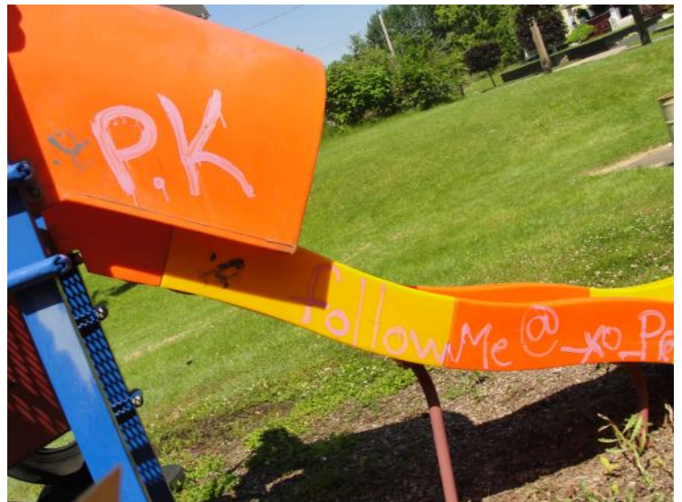
Playground equipment needs to be replaced.
